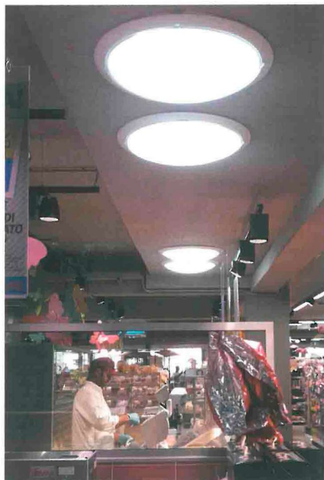
To optimize natural lighting, innovative light domes were deployed, which pass on sunlight through solar tubes.
